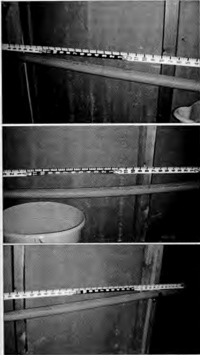
Figure 6 – Sagging of an installed CPVC pipe exposed to a mixture of water and bio-glycerin.
